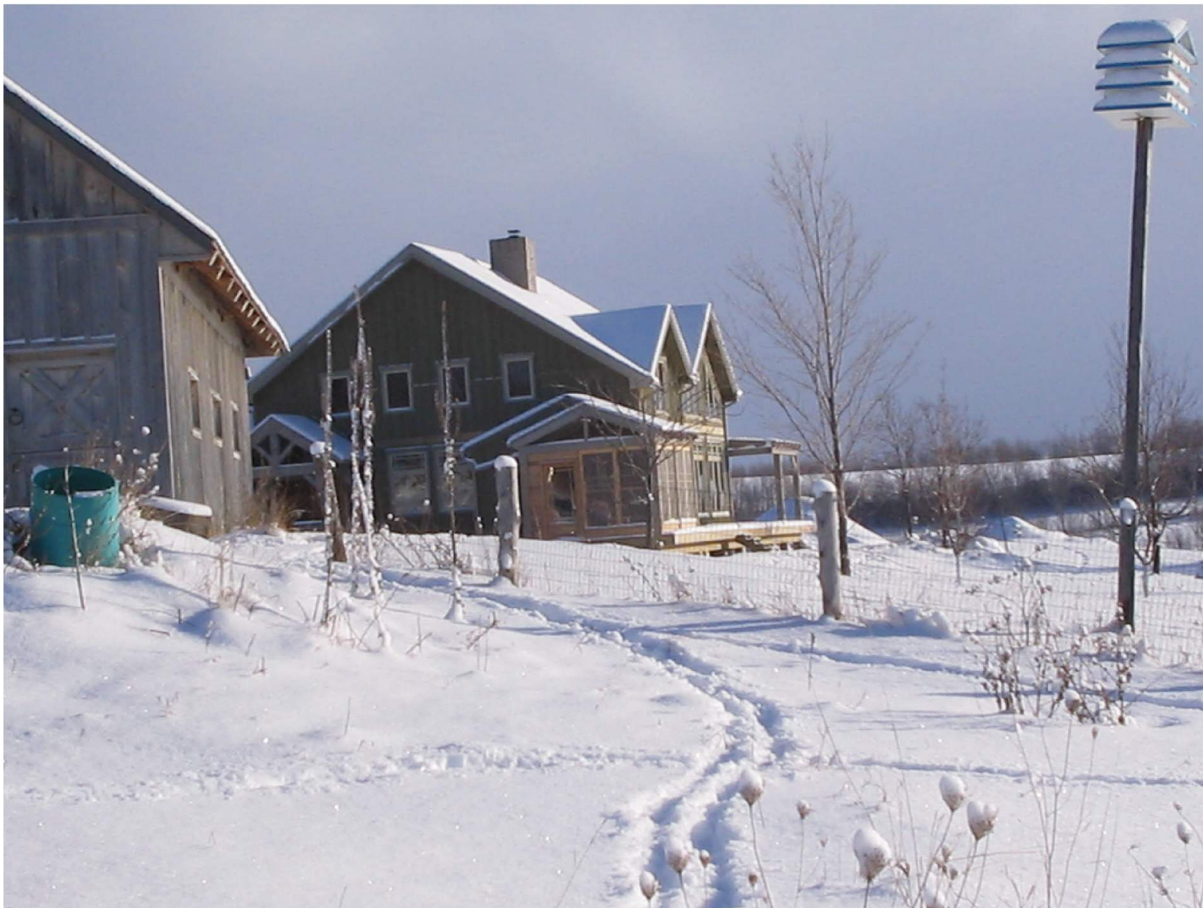
View of Frog's Hollow: Cedar shakes and siding, timbers and floor planks were sourced locally.
