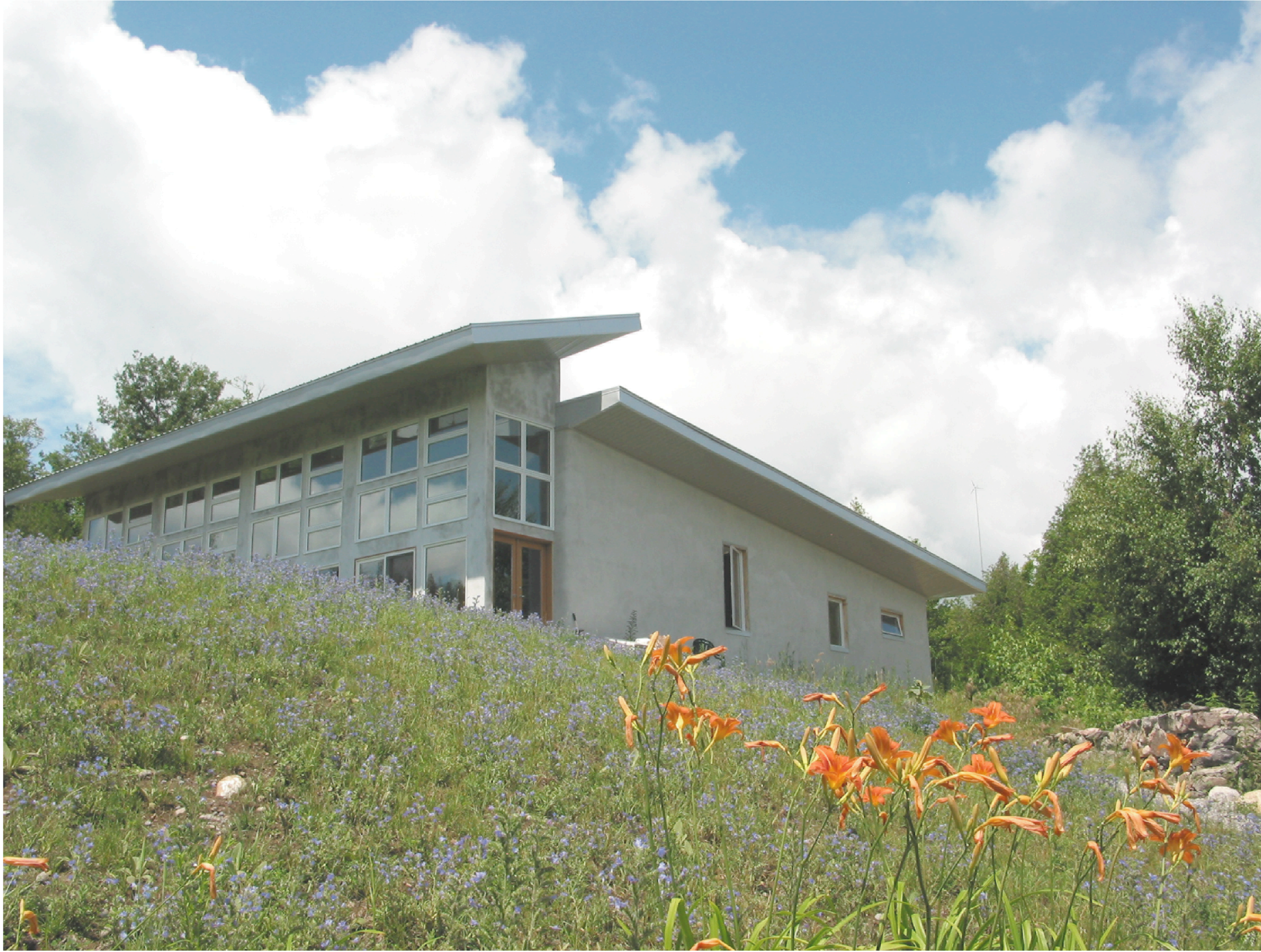
Hunter House was designed holistically to ensure that placement on the site, window-orientation, thermal mass, and innovative mechanical and electrical systems would work together most effectively.
