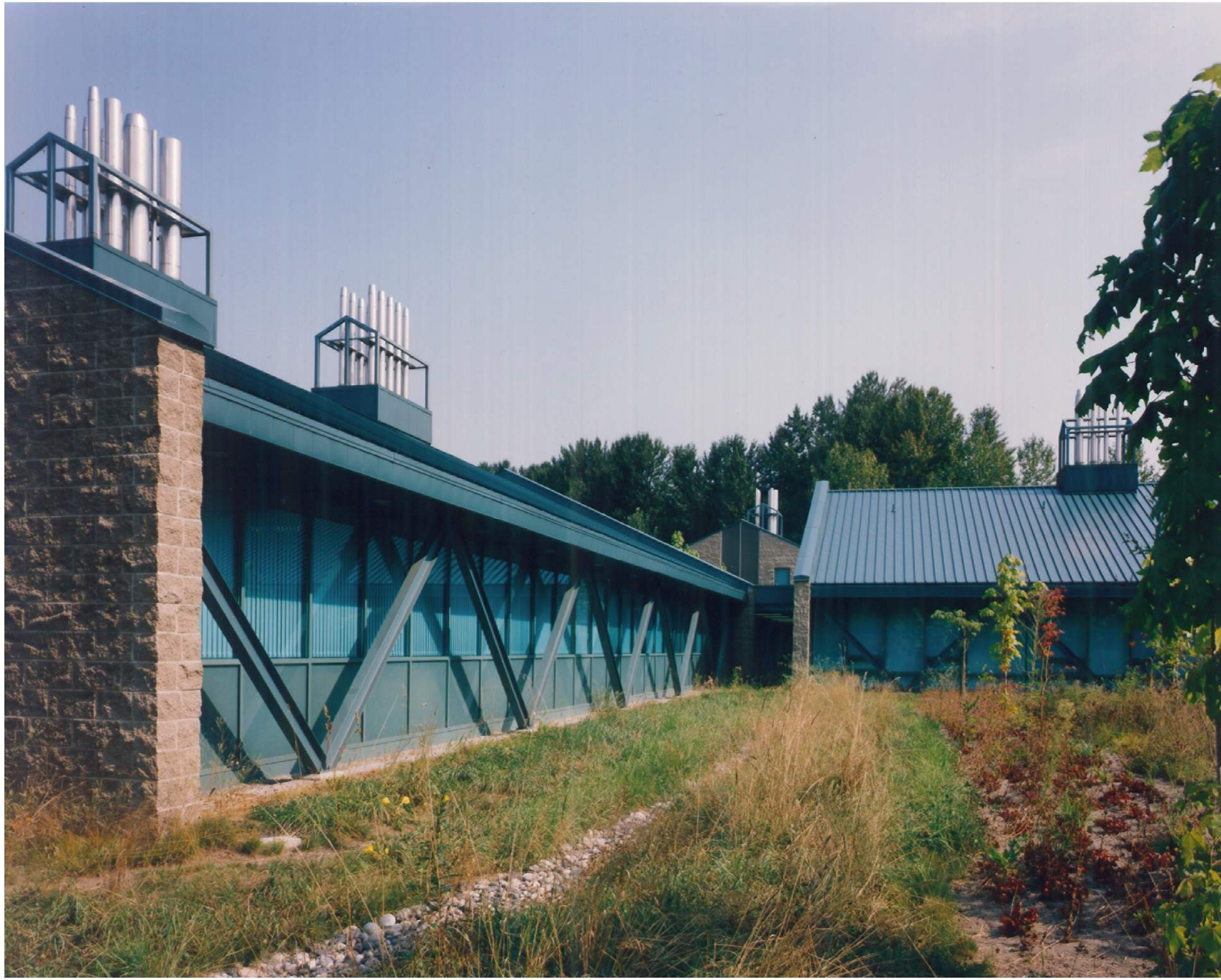
The buildings are designed as a series of linked pavilions to engage the surrounding landscape. An innovative exterior truss system supports the roof structure to provide a column-free laboratory environment.
